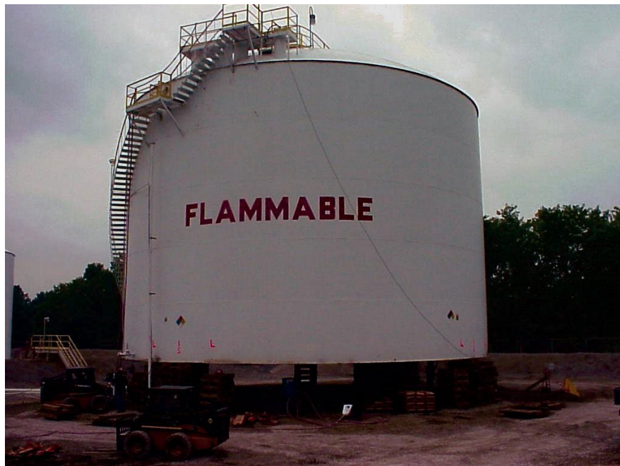
Figure 51—Tank Jacked Up for Repairing Pad
