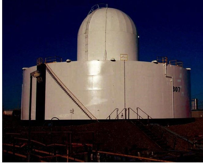
Figure C.9—Tank with Vapor Dome Roof
