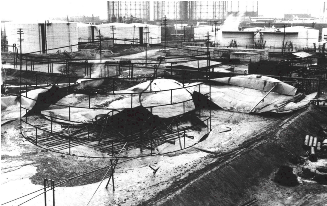
Figure 17—Extensive Destruction from Instantaneous Failure
