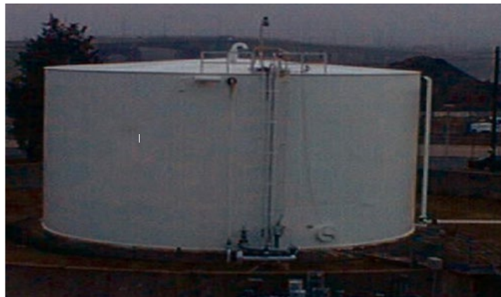
Figure 1—Fixed Cone Roof Tank
