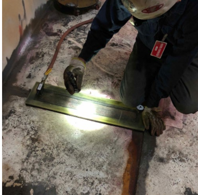
Figure 46—Vacuum Box Used to Test for Leaks
