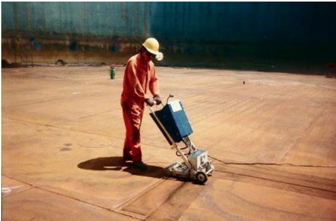
Figure A.2—Magnetic Flux Leakage Scanner
