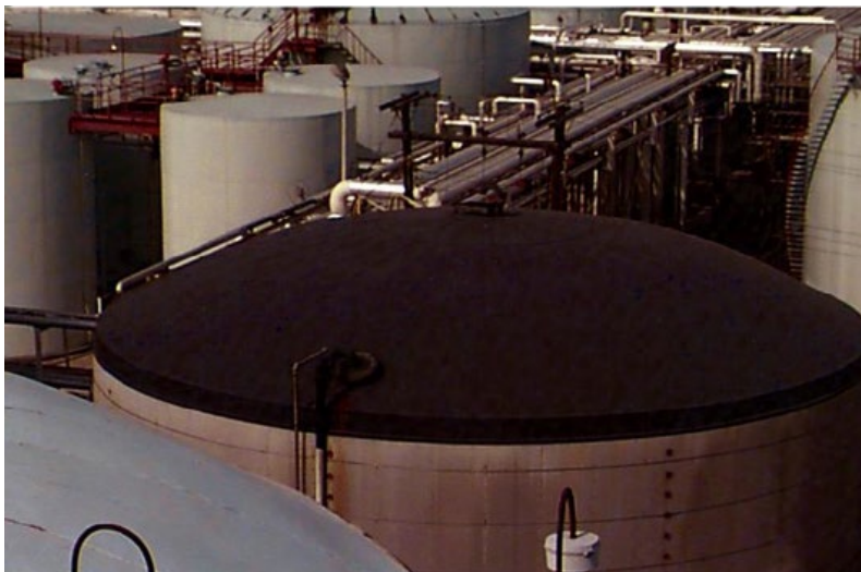
Figure 2—Self-supporting Dome Roof Tank
