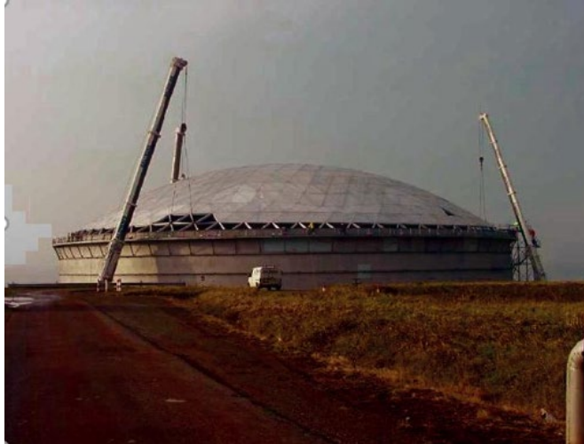
Figure 4—Self-supporting Aluminum (Geodesic) Dome Roof Tank
