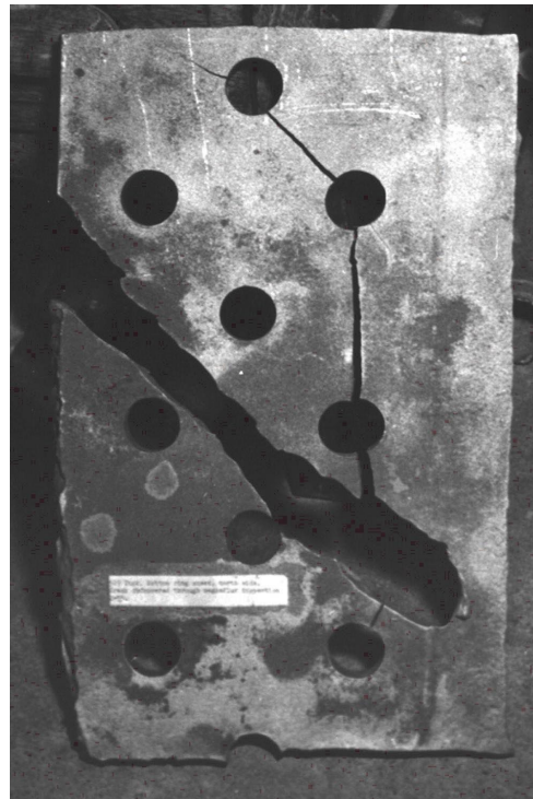
Figure 19—Cracks in Tank at Riveted Lap Joint to Tank Shell
